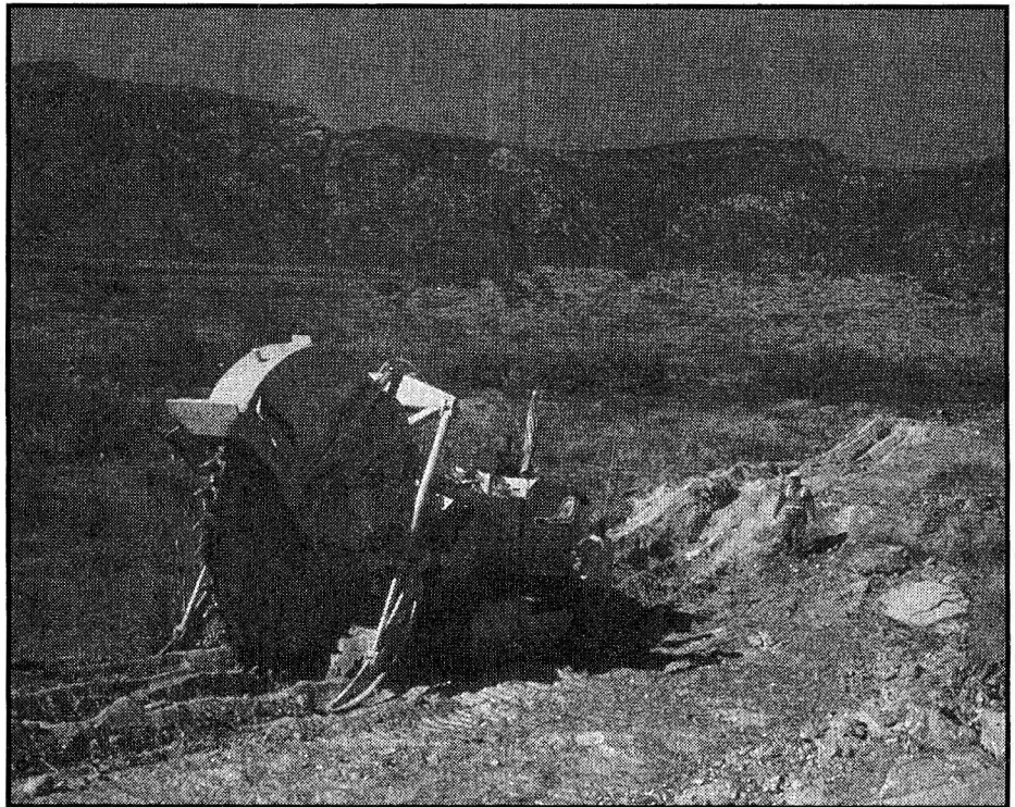
Men and machines cut a 23-mile long trench through desert habitat to lay the powerline.
