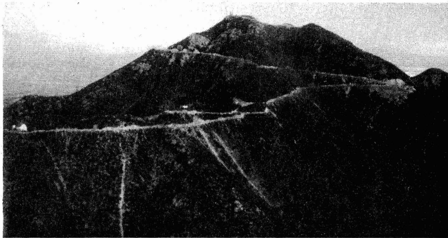
Erosion effects are clearly visible on this road built up Mount Hopkins in the Coronado National Forest. The road was cut to allow an astronomical observatory.
